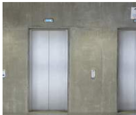
Exposed concrete lift core
