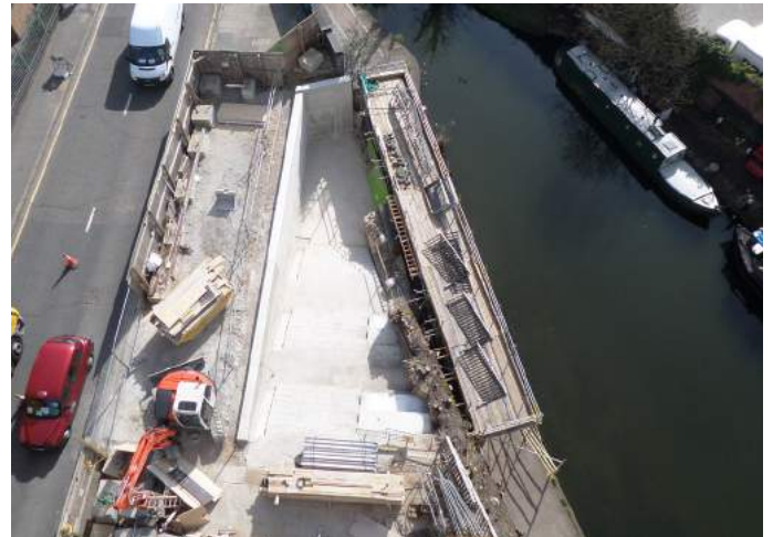
View of towpath stairs during construction
