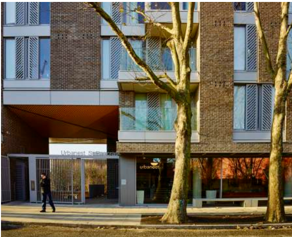
View of completed soffit
